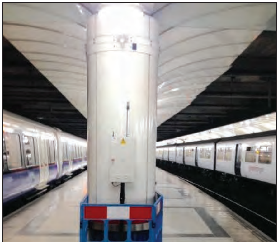
© Network Rail. Air quality monitoring kit on station platform.
