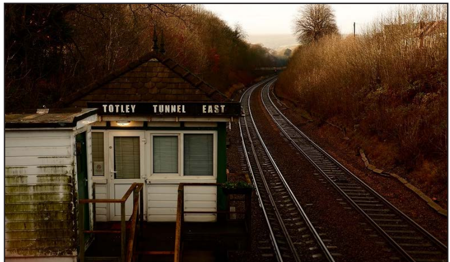
Totley Tunnel East signal box
