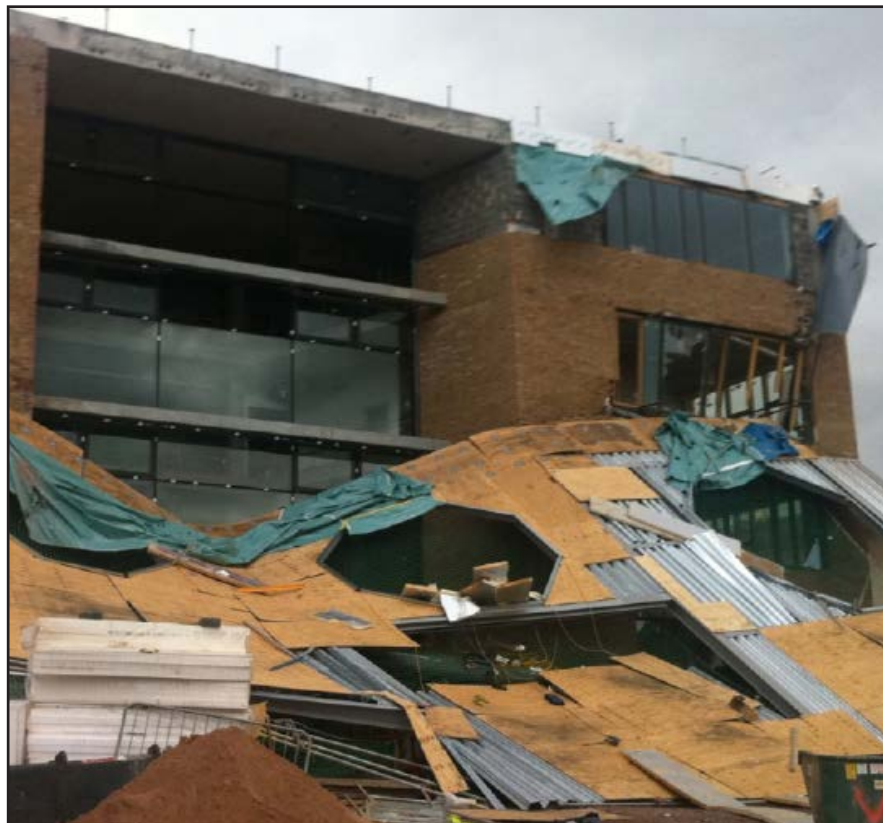
Collapse of the steel framed canopy. © Structural Safety
